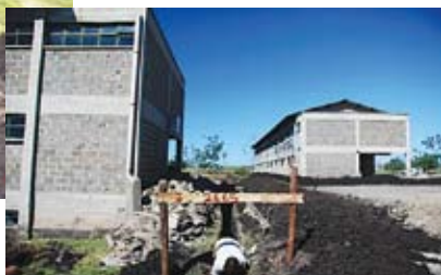
Basement retaining wall foundations
